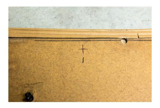
**STEP 8: Drill your mounting holes** Once you're confident that your marks are accurate it's time to drill. Take your drill and 1/8" bit and make your holes. We find it's easiest to press and rotate the bit against the panel (or use a centerpunch) to provide a divot to keep the drill aligned to your mark. Be conscious of what's on the other side of the panel—**don't drill into your table!** Take your time and hit your marks. Your patience will be rewarded with a clean installation.
