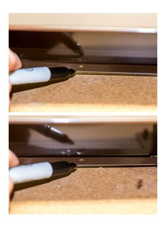
Here's an alternate method if you're having trouble making an accurate mark on the bottom two mounting holes. Mark a line on the panel along the bottom of the pocket. Mark the two hole locations above the holes in the pocket. Remove the pocket and measure from the bottom edge to the center of each hole. Then measure the same distance from the line you made on your panel and mark the hole. Reinstall the pocket to verify your marks. See the picture below for reference.
