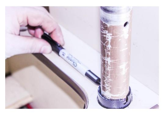
9. Remove the table and leg from the van, and position somewhere that makes it is easy to drill the hole. (Removing the table from the support leg will help).
