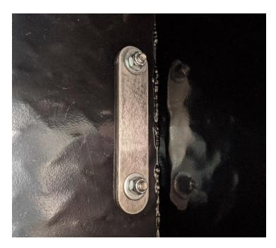
8. **(For the 24 1/8" wide boxes only)** The last step of the installation is to drill through the outside gussets and into the storage box. Then install and tighten the remaining (4) ¼" Carriage bolts, (4) ¼" washers, and (4) ¼" Nylock nuts. Clean up the drill shavings using a vacuum.
