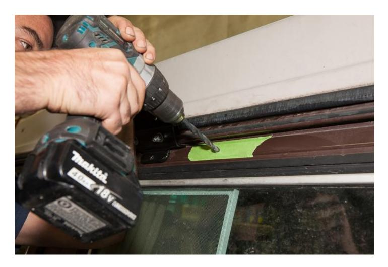
Take one of the **Rivet Nuts** from **Hardware Package B** in slide it into the hole you just drilled. The shoulder of the Rivet Nut should be facing outwards.
